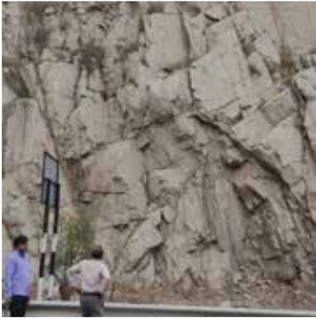
2km road ways hillslope, Slope Stability Survey
