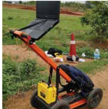
Ground Penetrating Rada survey for electrical line
