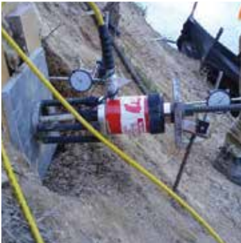
Pull Out Test Performed at Airoli, Interlink Tunnel
