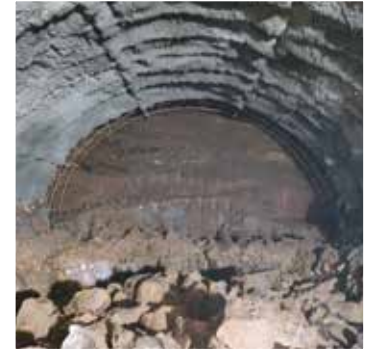
Geological Face Mapping of NATM Tunnel for Design & Construction
